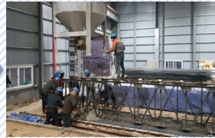
③ "A"판넬 콘크리트타설
