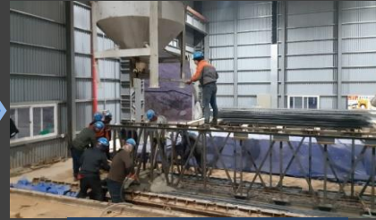
③ "A"판넬 콘크리트타설
